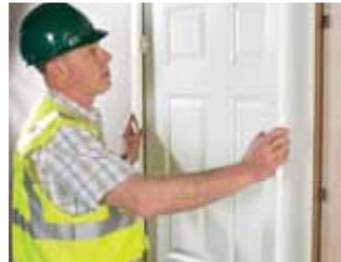
Firmly push the architrave into the locating groove in the door lining. Pinning is not necessary. If required, paint the door, frame and architrave. Handles (not supplied) may now be fitted and the installation is complete.
