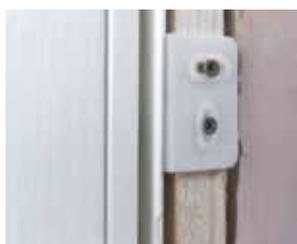
It is recommended that a timber stud lining frame should be fitted within the wall aperture prior to commencing installation of SpeedSet Plus doorsets. To ensure compatibility with standard unit frame sizes, dimensional allowance should be made for the thickness of this sub frame. (See back page).
