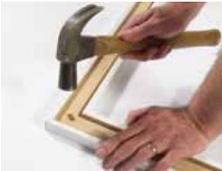
To prevent damage, lay the matched architrave components face down on a flat, clean surface. Butt the joints together and fix by carefully tapping the 'butterfly' clip supplied into the pre-cut slot. After assembly check the fit of the architrave into the groove on the door frame before proceeding to Step 9.
