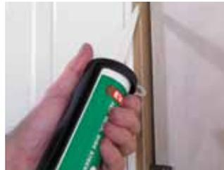
Apply a good quality gap filling adhesive into the architrave location groove in the door lining. Take care not to apply too much adhesive as this may cause difficulty when fitting the architrave. To avoid staining, excess adhesive must be removed immediately. Always follow the adhesive manufacturers instructions.
