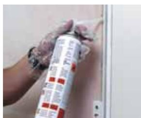
At Step 6: In addition, fill any gap between the frame and the wall with fire retardant foam or other suitable fire blocking material.
