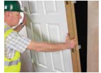
If one is fitted, carefully remove the disposable transit brace from the bottom of the door frame. Offer the doorset into the wall opening, plastic bracket side first, ensuring plastic brackets are extended. Push the doorset into the wall opening until the rigid steel brackets make contact with the wall. SpeedSet Plus is designed to give a 15mm gap under the door. If a greater gap is required lift the frame using packers. If a smaller gap is required trim the bottom of the lining.
