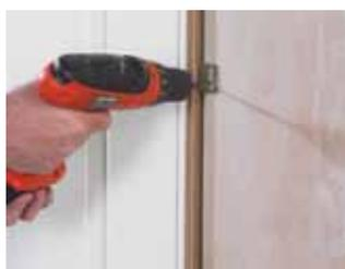
Position the doorset vertically and centrally in the wall opening. Fix the brackets to the wall using the 40mm screws by inserting through the horizontal bracket slots. If necessary use packers to position the door set.
