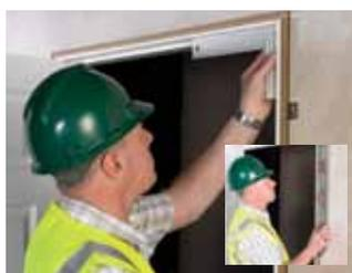
Check that the frame is plumb, square and securely fixed, also that the door operates freely. Adjust if necessary. If the latched door 'rattles', this can be eliminated by bending the tab in the latch keep.
