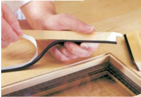
Fitting FD30 Glazing System
